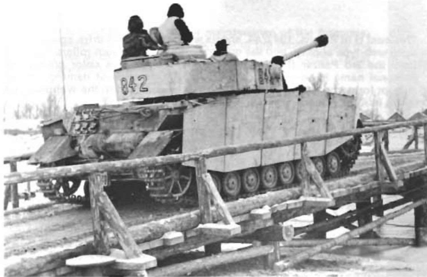
This relatively new ausf H traveling over a log bridge in Russia has unusual side skirts in that the "standard" system of brackets, rails, and teeth are used to hang the skirts, yet the front three sections have the edge cutouts and central holes used with the older hook-type design. (Bundesarchiv)
