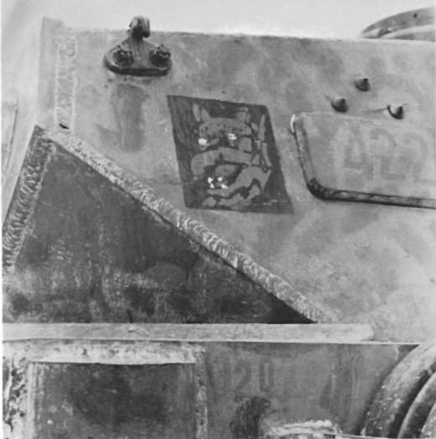
This close-up of another vehicle from the same unit shows very clearly the structural welds in the turret and hull fittings. The mottling on this vehicle has been brushed on rather than sprayed. (Bundesarchiv)
