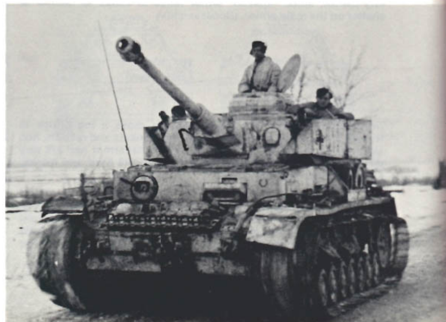
(Above Right) This late production PzKpfw IV ausf G in Russia resembles very closely the later ausf H. This vehicle still has the folding radio antenna and trough and the split cupola hatches, along with the L/43 KwK 40. However, it also has turret skirting and the added 30mm frontal and nose armor. This shot also shows very clearly the wide "Ostkettens" ("eastern tracks") used in Russia because of the poor weather and terrain. Note the bogey truck on the glacis and the gap left by its removal. (Bundesarchiv)
