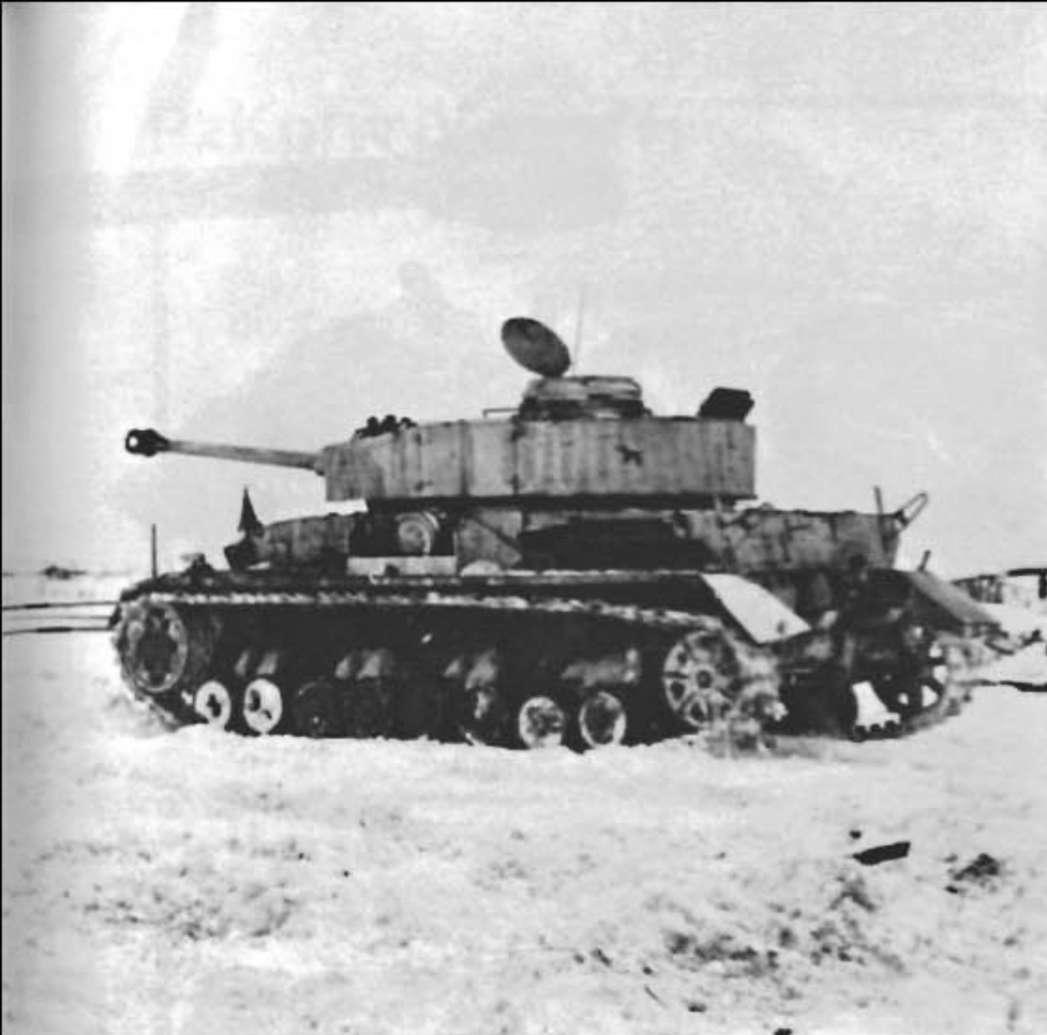
An ausf H, not fitted with hull skirting or brackets. The crew has sprayed white in a vertical wave pattern over the turret skirts. The chassis was not usually repainted. (Bundesarchiv)
